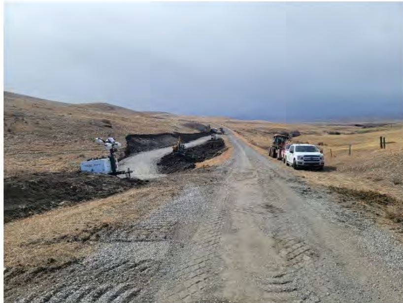
March 20, 2026 Looking Southwest, completed detour road
