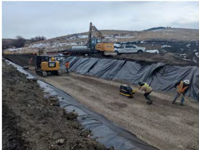
March 28, 2026 Backfilling and base packing underway. 5-10 passes needed.
