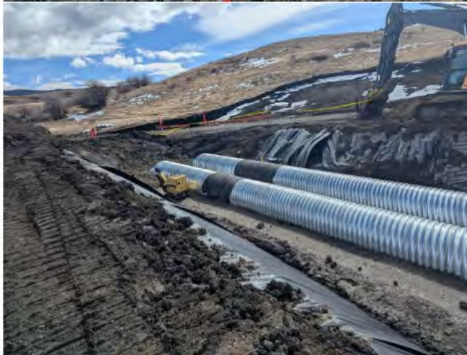
April 3, 2026 Pipes bolted together and backfilling had begun.
