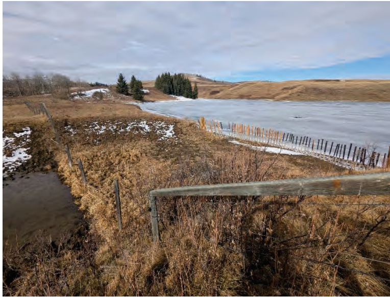
Figure 3: Flow Obstructions at Spillway Inlet
