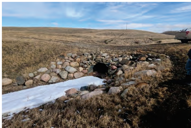
Figure 4: Upstream Dam Access Road Culvert Crossing (Sta. 0+234)
