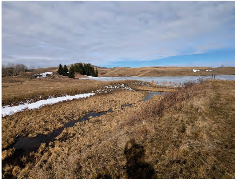
Figure 2: Vegetation Grown in Spillway Flat Section
