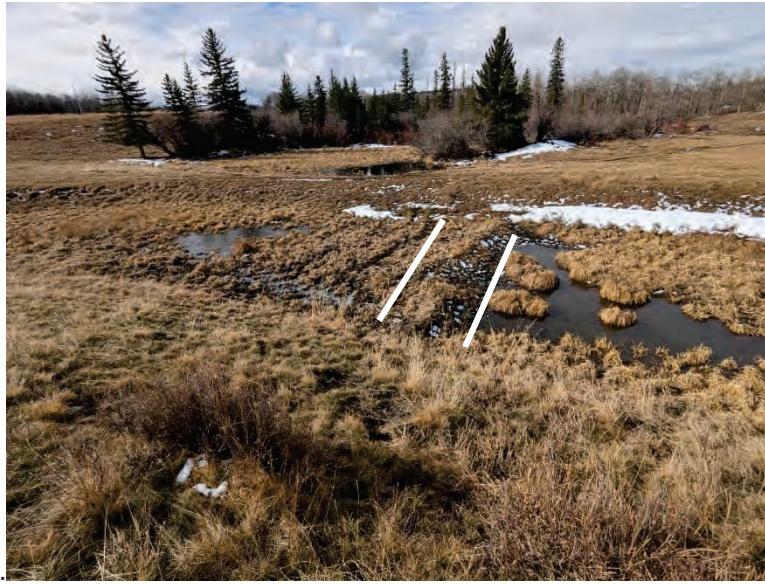
Figure 1: Grassed Weir at Sta. 0+050 Backing Up Water
