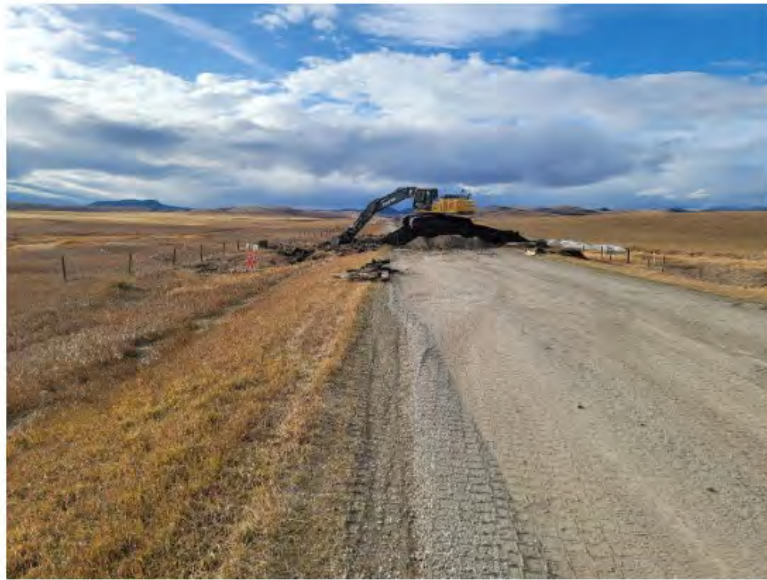
November 12, 2025 Excavation and Bridge Removal
