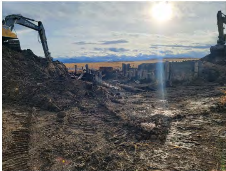
November 12, 2025 Excavation and Bridge Removal, looking south
