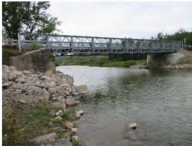
5. Looking north along D/S profile. Previous massive abutments and wingwalls left in place.
