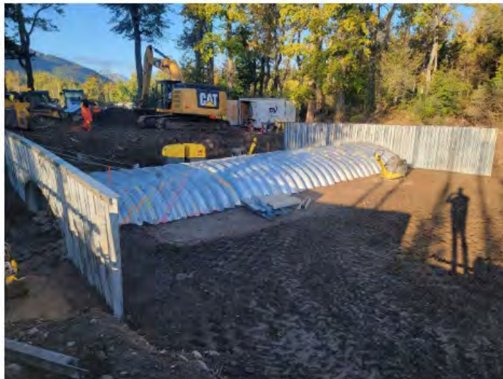
September 23, 2025 Roadway Structural Backfill
