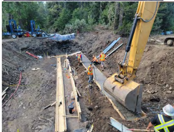
August 15, 2025 1st footing concrete pour
