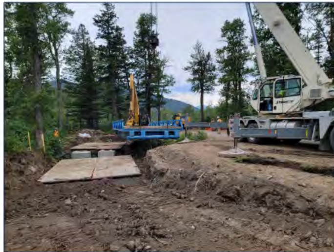
August 6 2025 Detour bridge being placed
